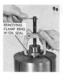
turning them slowly and equally to prevent breakage of the clamp ring. Then the three short cap screws may be removed. (Refer to photo 7a for determining long and short bolts before loosening any bolts.)
